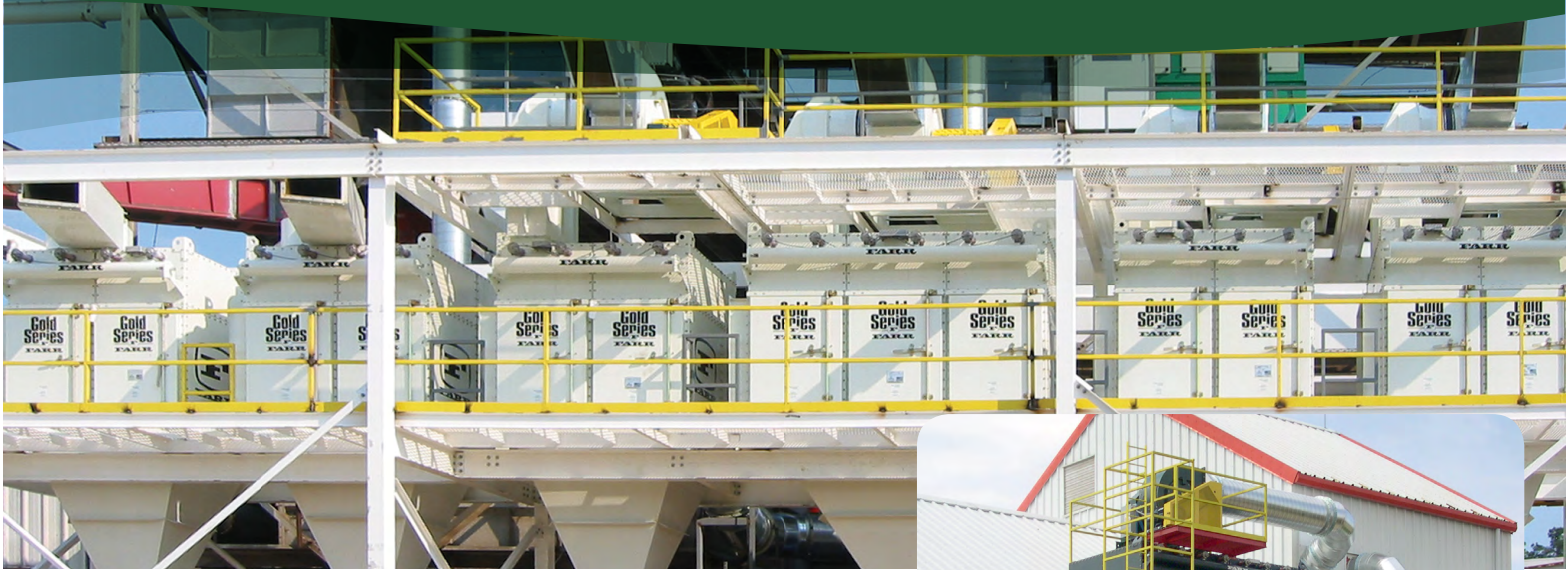
Multiple FGS Dust Collectors on Corn Processing
